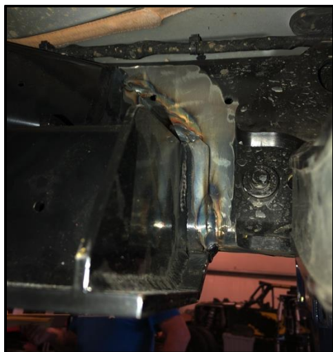
Back Side Weld
