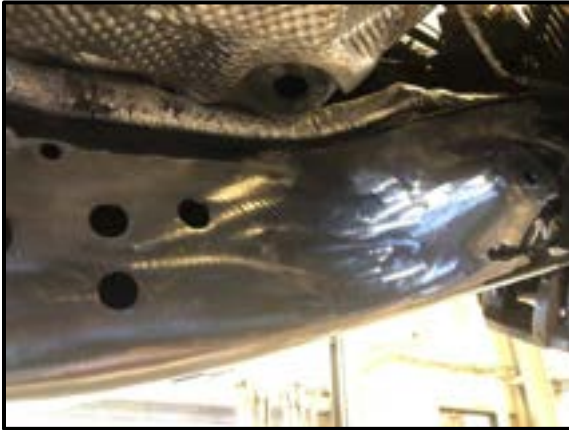
Driver's Side Front Frame Rail
