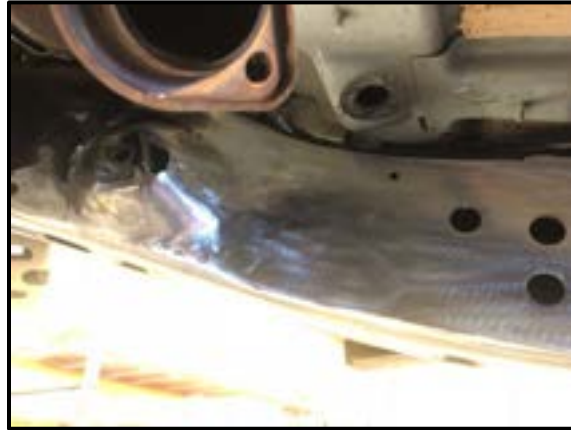
Pass's Side Front Frame Rail
