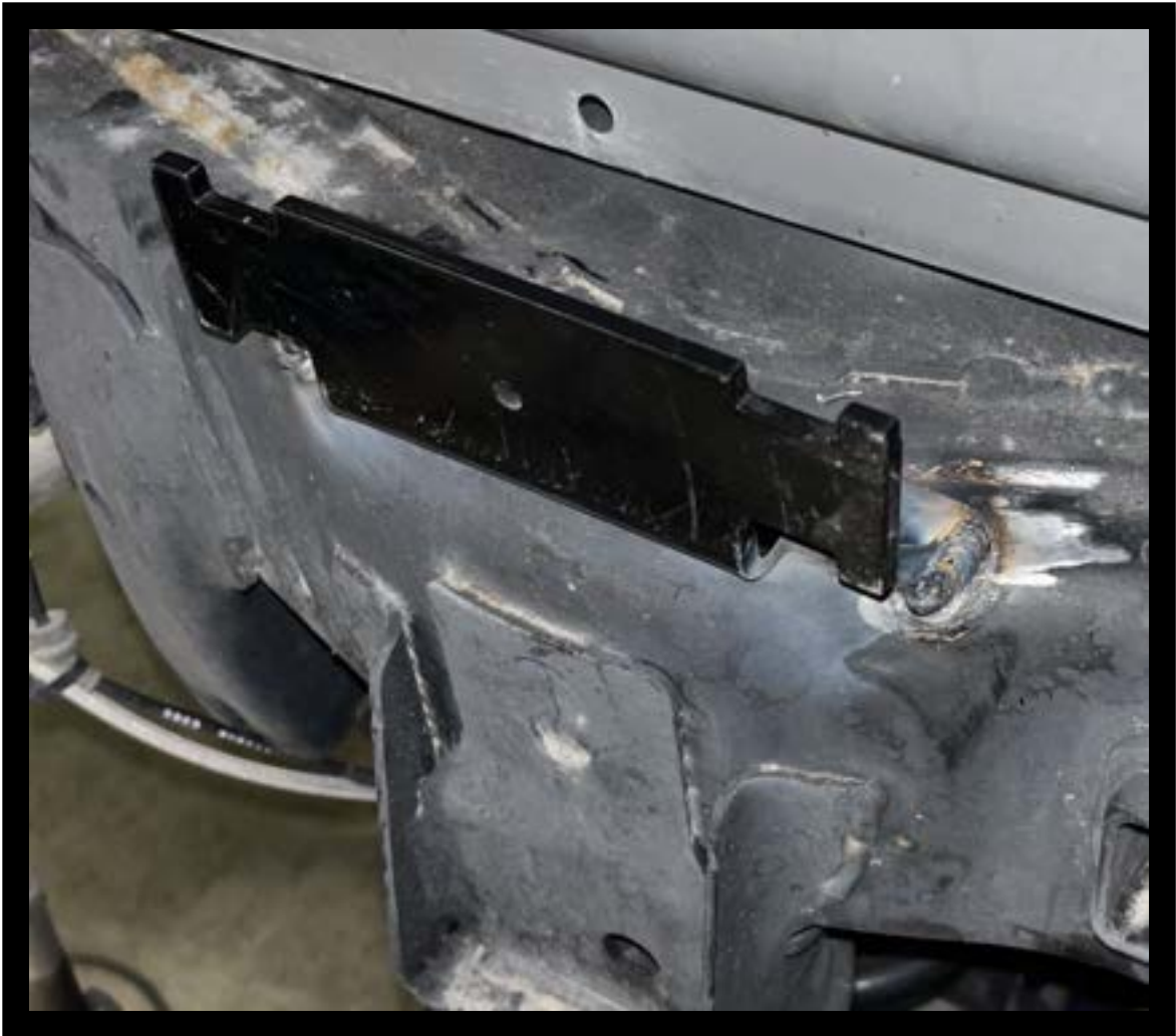
Ressy Mount Welded to the Frame
