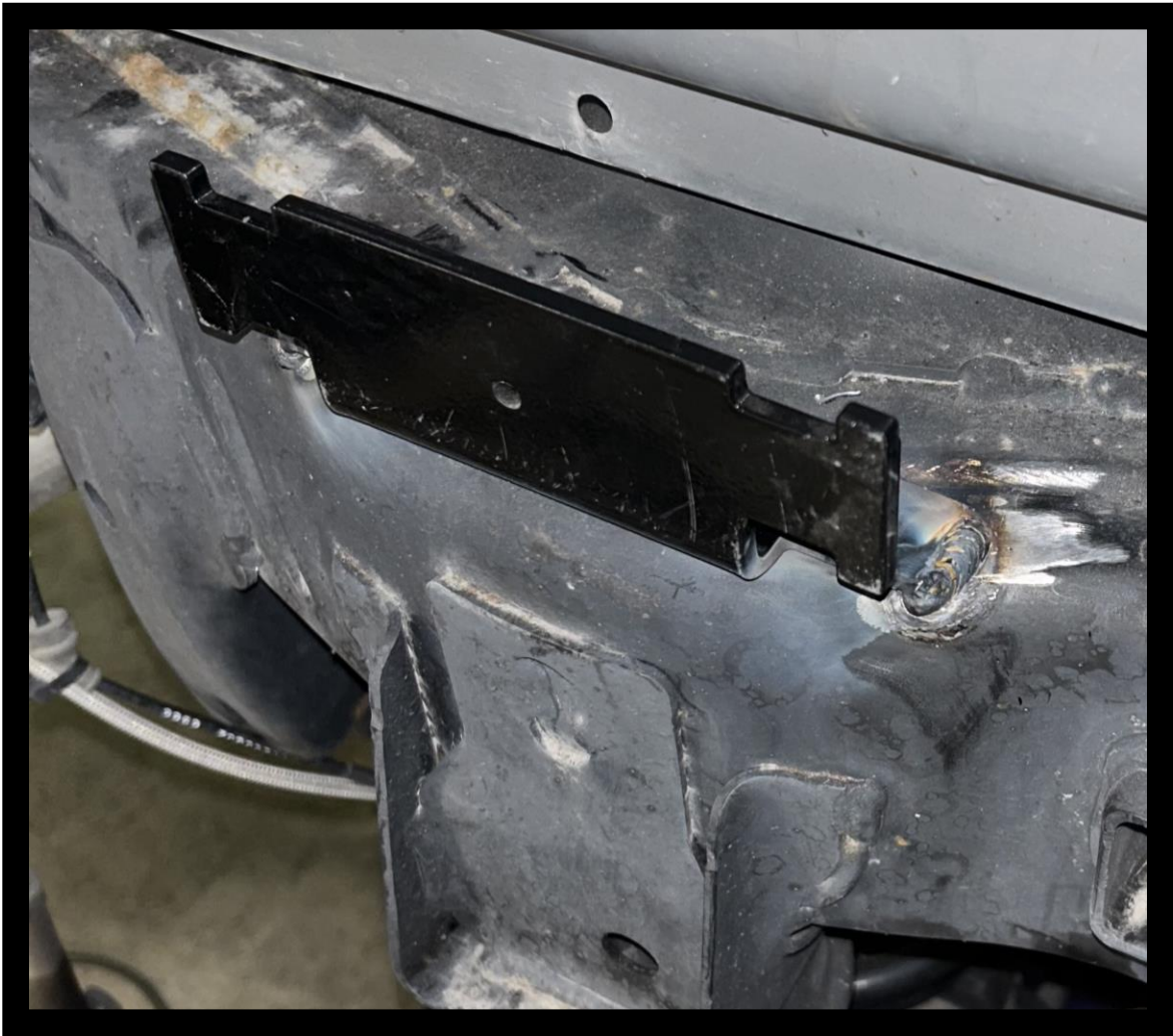
Ressy Mount Welded to the Frame
